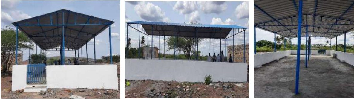
Constructed Iron shed at Renuka yallamma temple Kalva village.
